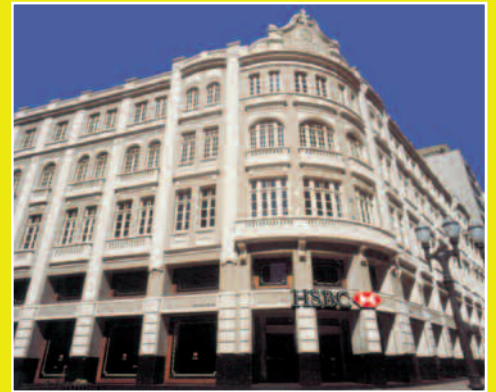
HSBC Bank Brazil's headquarters building in Curitiba, Brazil
